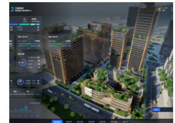
iBUILDING-Douyin Group Smart Park Operation and Management Center
